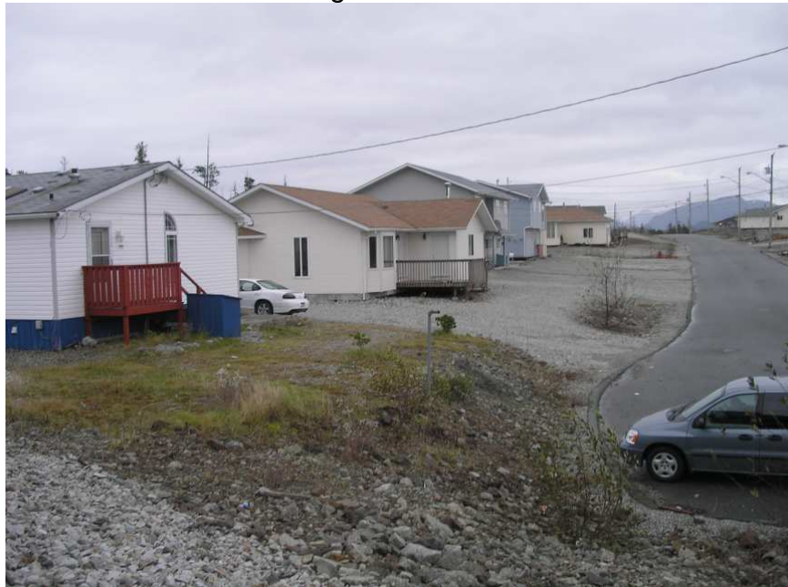
Figure 4. New developments at north end of village with low amounts of combustibile material and good forest set backs.
