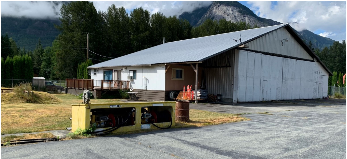
Existing Fuel Cabinet – To Be Removed
