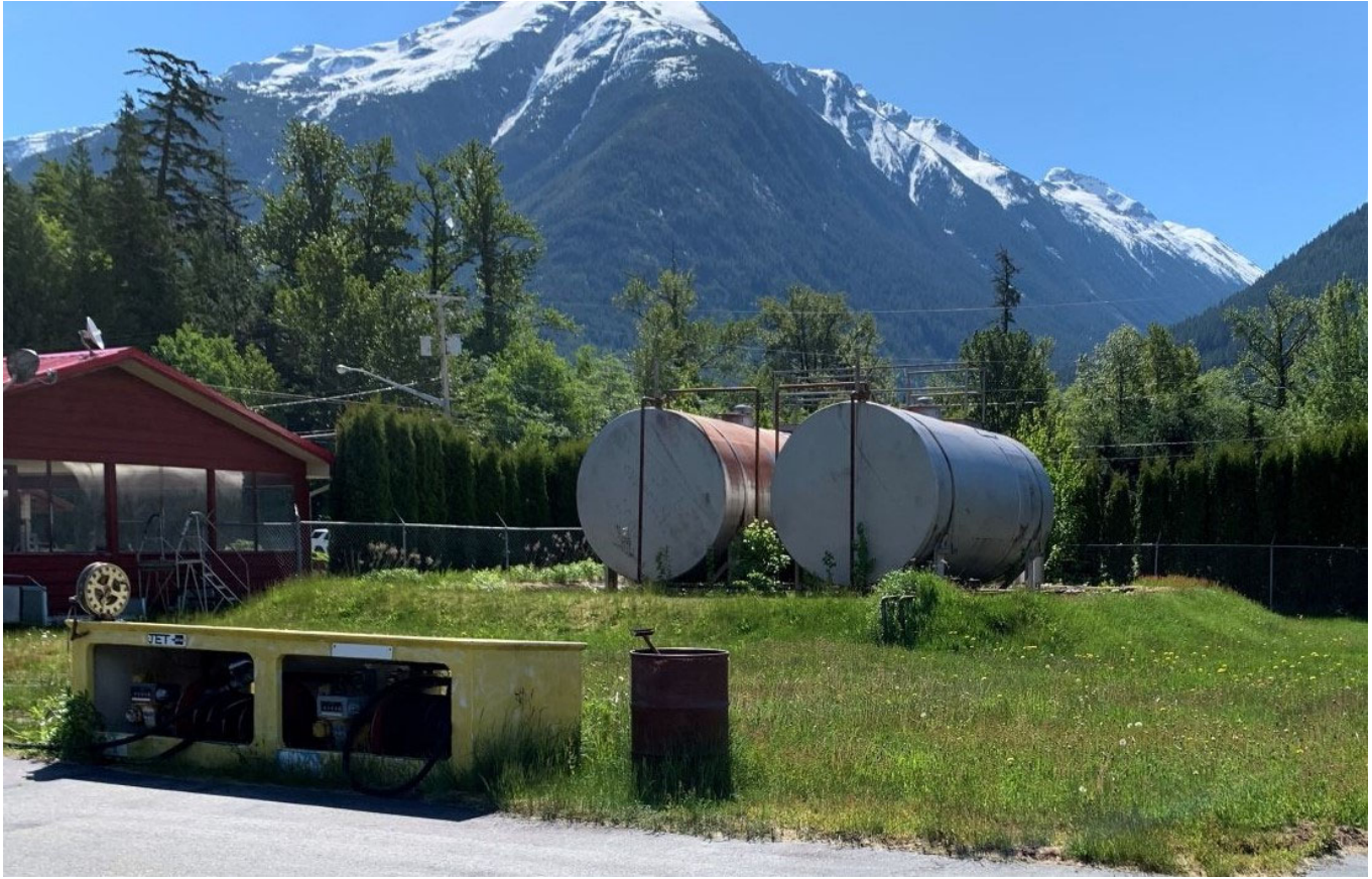
Existing Fuel Cabinet and Tanks – To Be Removed
