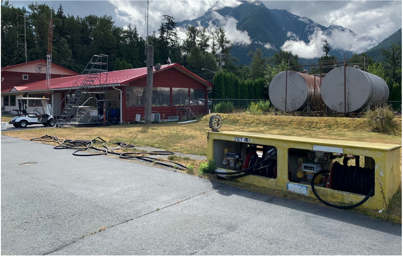
Existing Fuel System – To Be Removed
