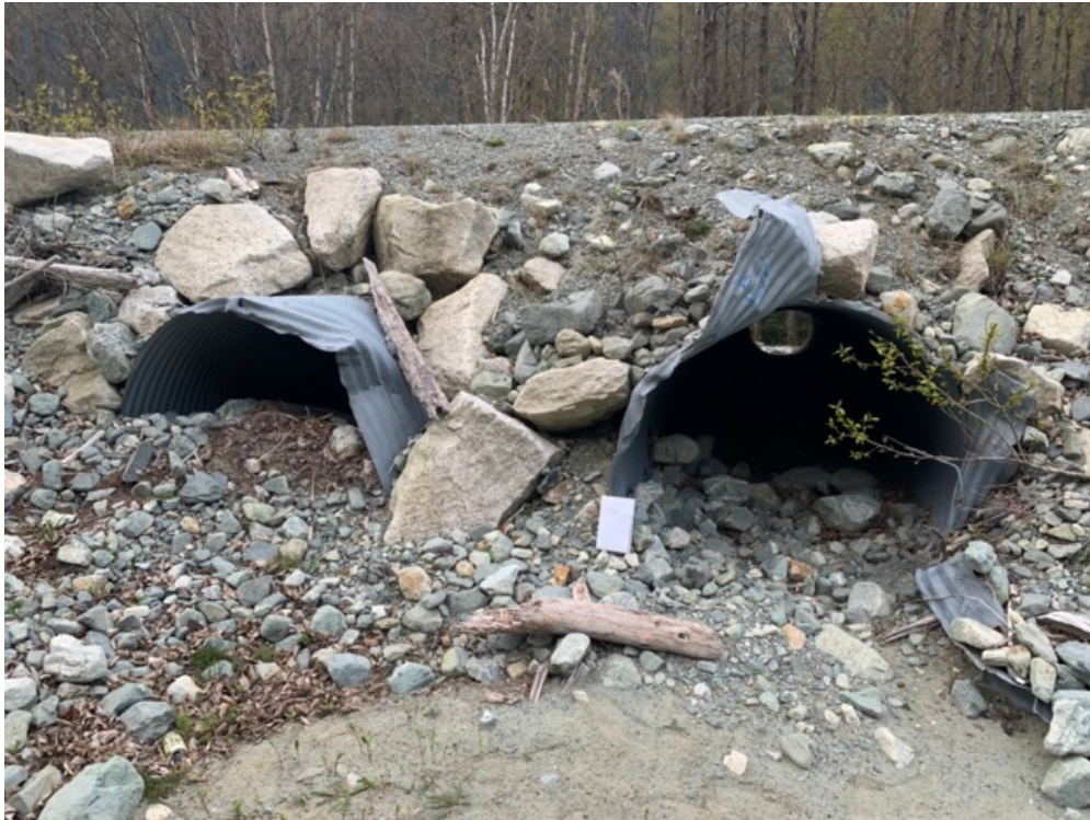
Photo 9 - East culverts inlet blockages
