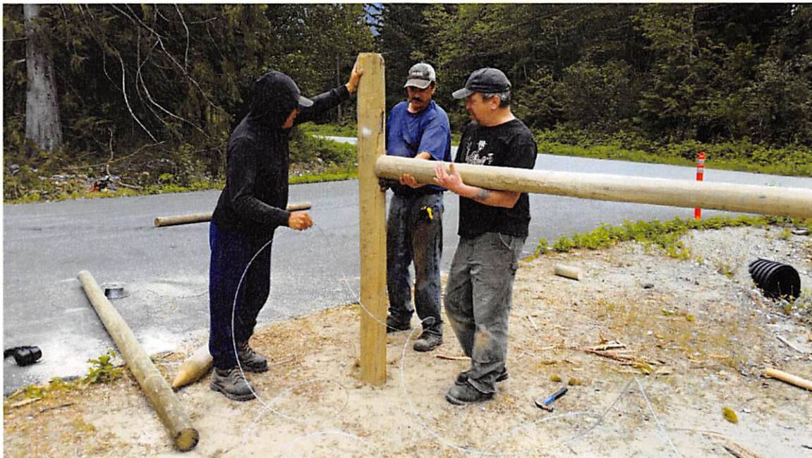
Photo: H-Brace construction at North gate entrance.
