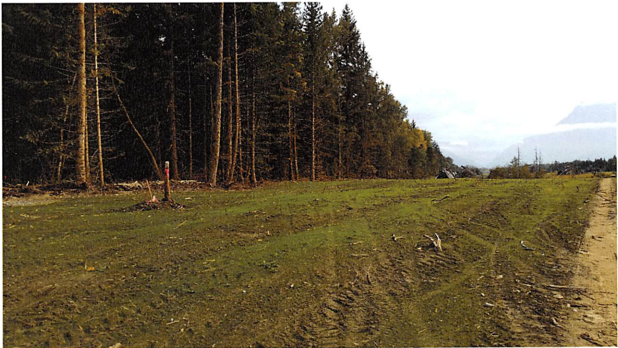
Photo: Private land portions on the northwest end have been cleared, raked, rotovated and seeded.
