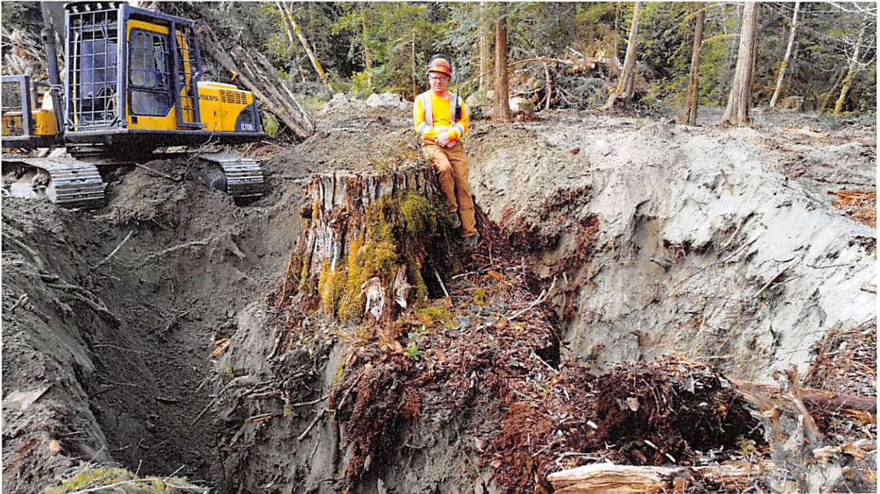
Photo 1: Large Cottonwood stump being dug out on the west end.
