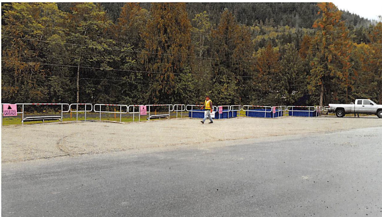
Photo: New drop off area for household garbage, metals, construction debris and wood waste.
