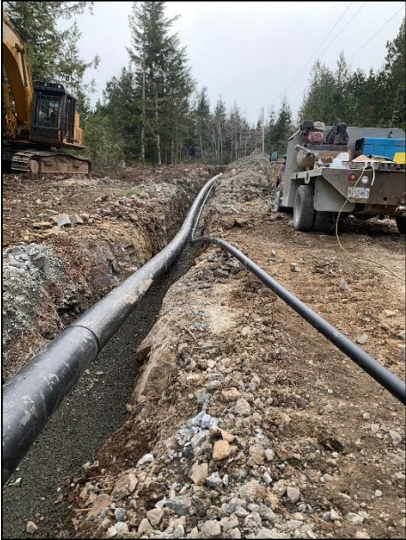
Reservoir Supply / Distribution Pipes
