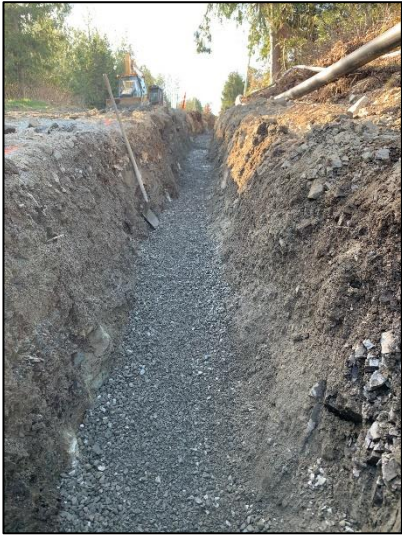
Trench / Pipe Bedding on Airport Road
