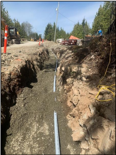
Reservoir Signal Cable Conduit
