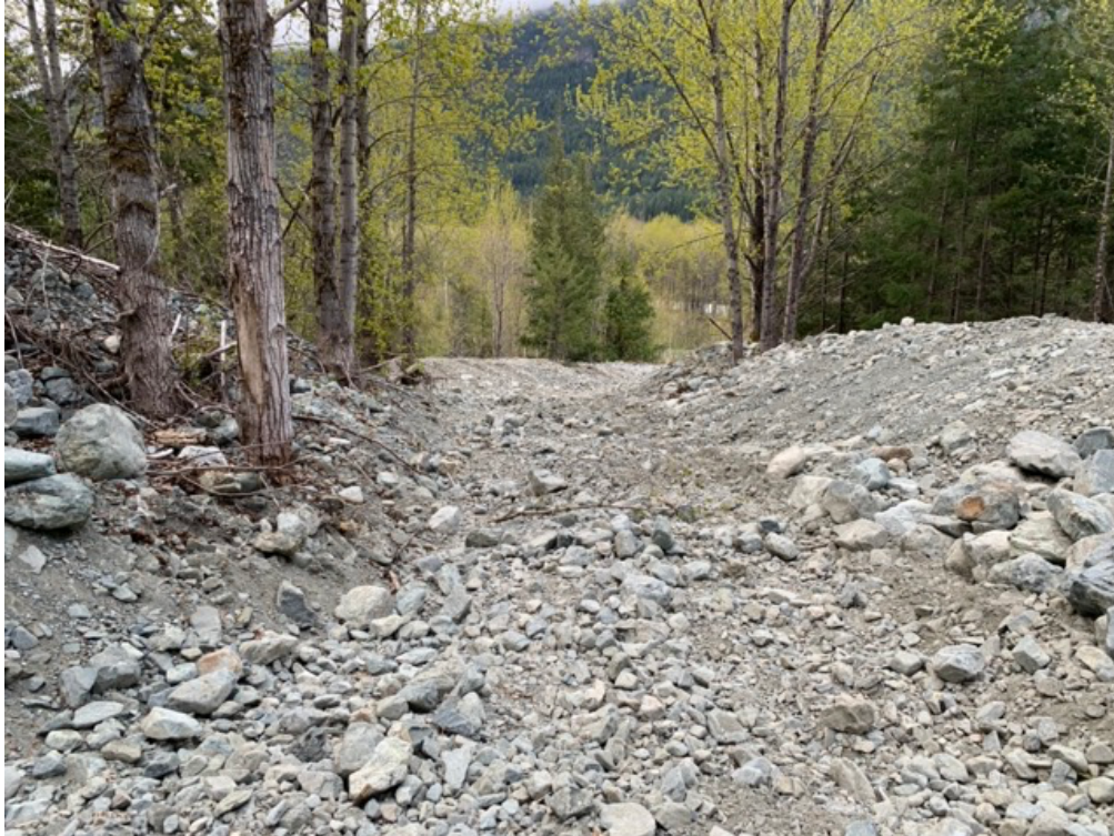
Photo 5 - West Channel looking d/s
