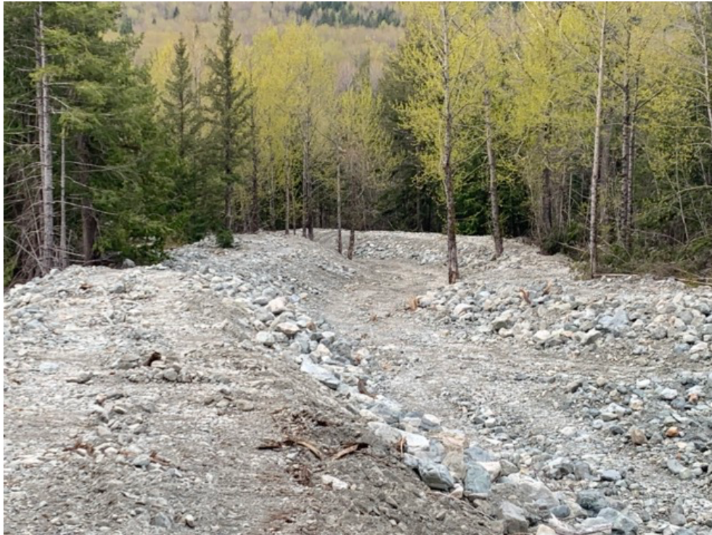
Photo 3 - Upper west channel looking d/s
