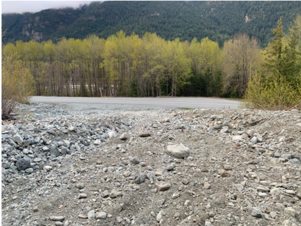
Photo 7 - End of West Channel berm and developed debris basin
