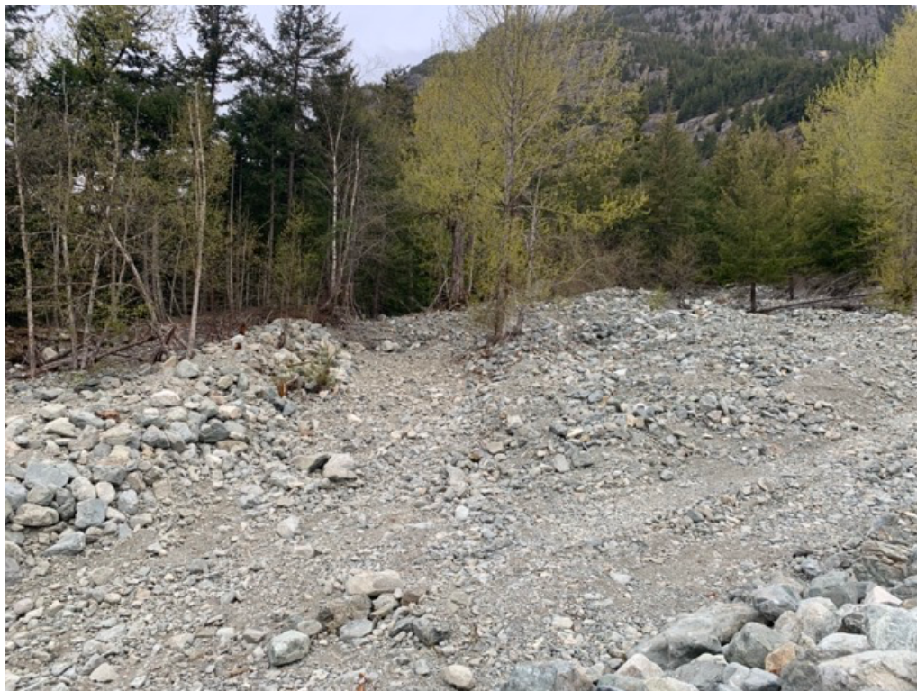
Photo 2 - Extension of west berm to cutoff avulsion point
