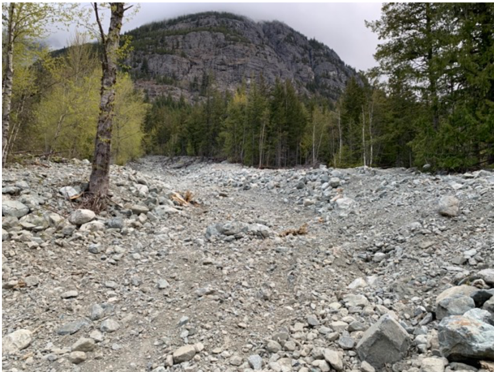
Photo 4 - West Channel looking u/s from end of East Channel cutoff
