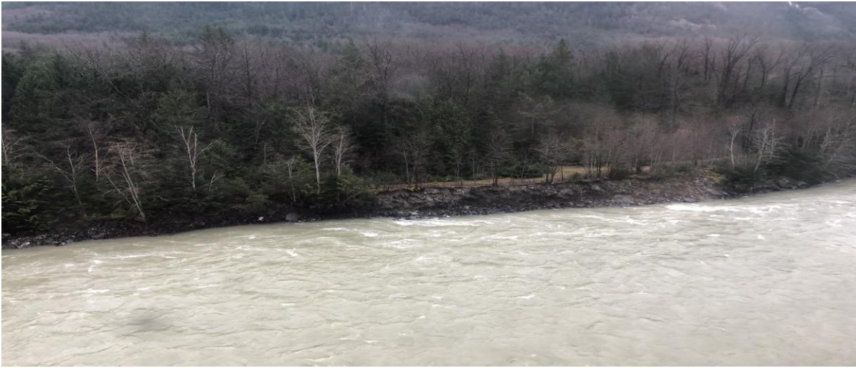
Fig 2 Upper Hagensborg Dike, Bank Erosion – Left Bank Bella Coola River
