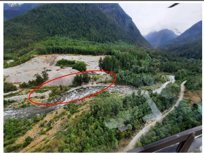
Phot 6: Right bank rip rap of Thorsen Creek remained intact with little or no obviously new erosion of the right bank upstream of the rip rap works observed.
