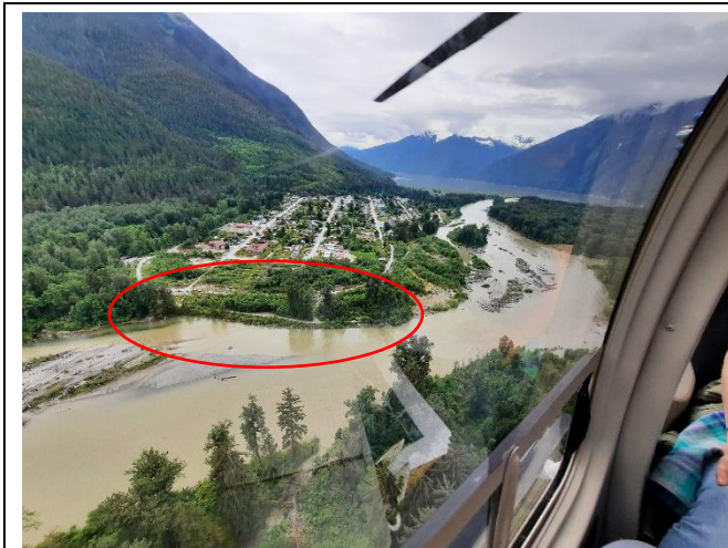
Photo 3: Left bank rip rap at Bella Coola townsite. No observation of water cresting the river-side dike and offset dike observed intact and unaltered.
