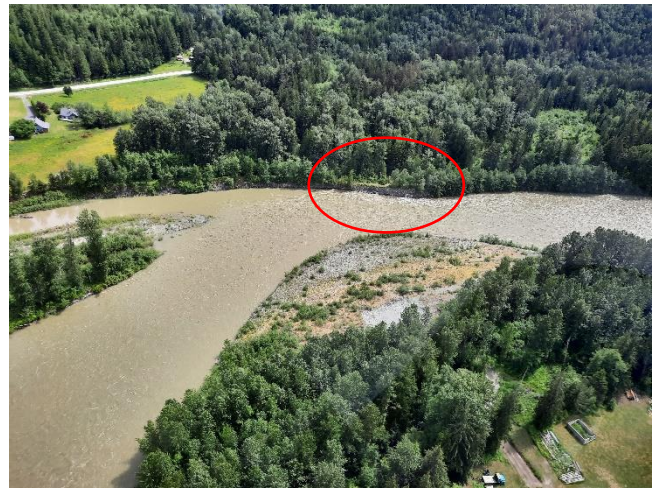
Photo 11: Area of possible past-recent erosion on left bank of Bella Coola River at Upper Hagensborg Dike. Undetermined if associated with June 16 rainfall.
