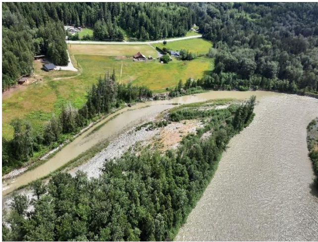
Photo 10: Upstream areas of Upper Hagensborg Dike now adjacent to a side channel of the Bella Coola River.
