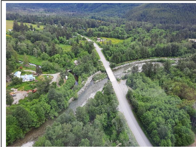
Photo 5: View east over Thorsen Creek Bridge. Bedload at bridge appeared unchanged from before June 16, 2022.
