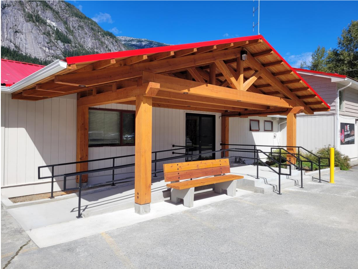
Photo: New Timber Frame Entrance to Bella Coola Airport Terminal. Completed August 2022. Photo Credit: Ken McIlwain
