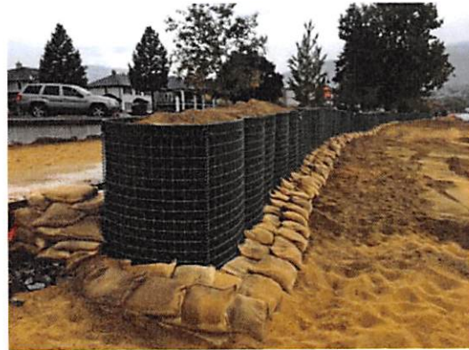
GABION BASKETS AND SANDBAGS
