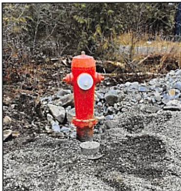
New Hydrant on Airport Road
