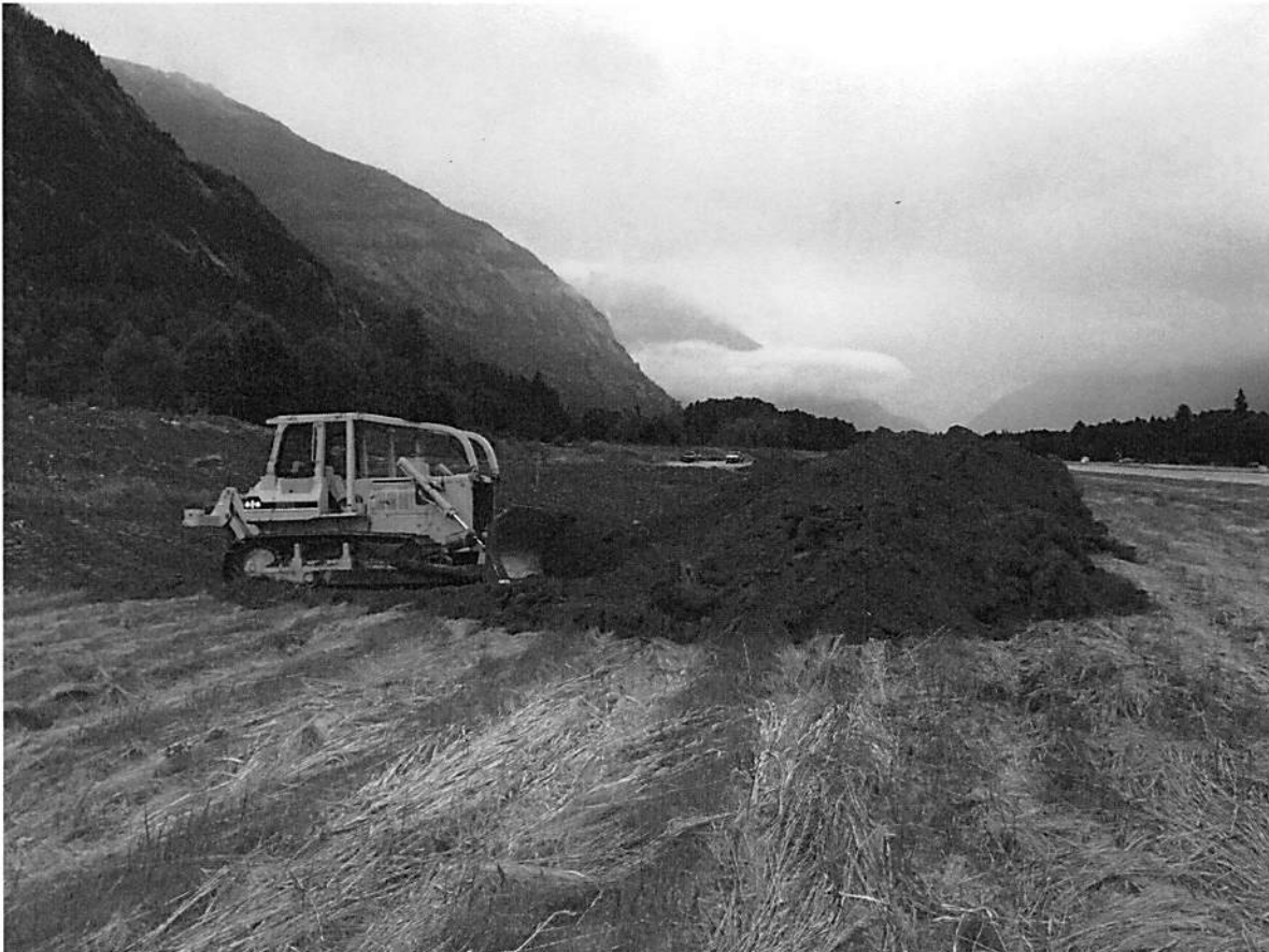
Photo: Stripping topsoil prior to burying gravel from the berm.
