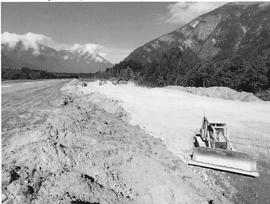
Photo: Spreading berm material in spoil area. Stripped top soil has since be reapplied.
