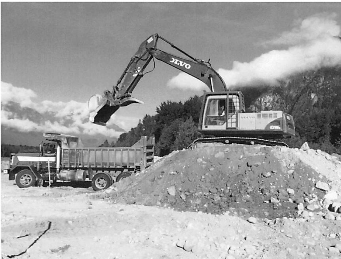
Photo: Trucking eastern portion of berm to spoil site for disposal.
