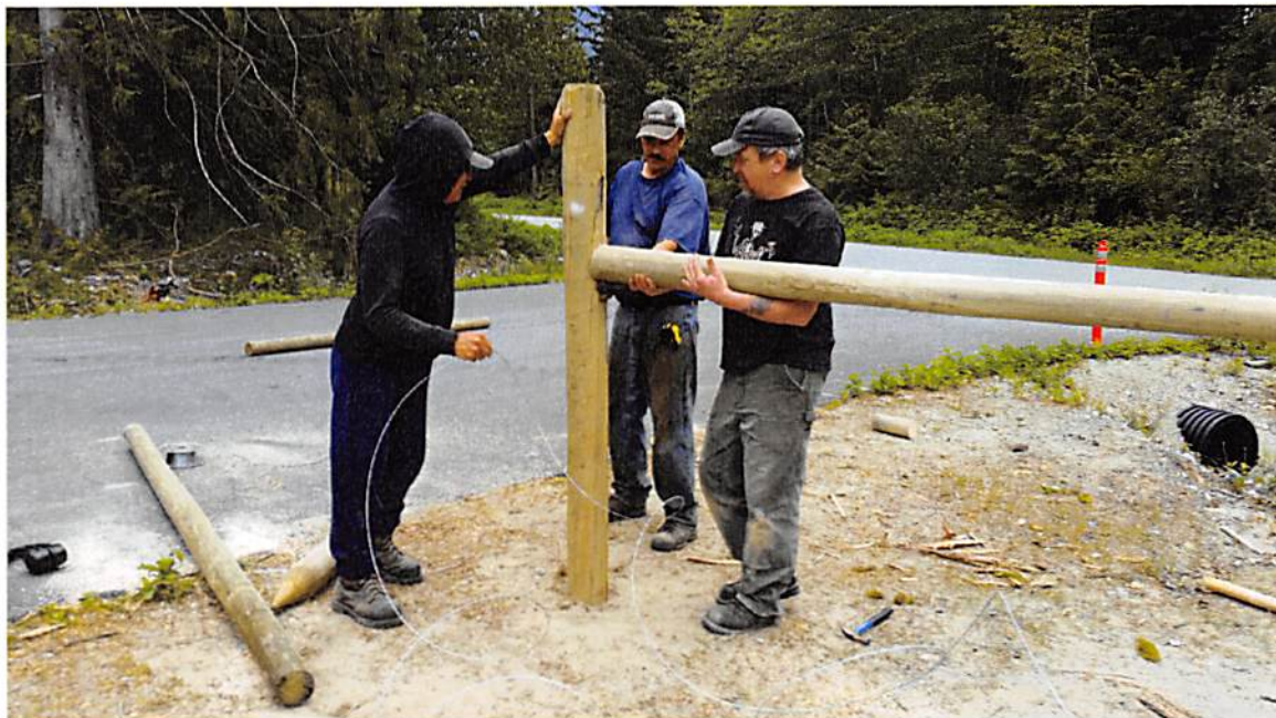
Photo: H-Brace construction at North gate entrance.
