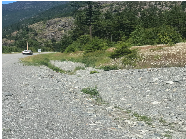
Figure 3 – West Culvert (June 2021)
