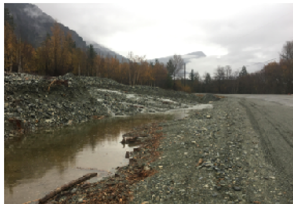
Figure 6 – Ratcliff Creek near East Culvert (Oct 2020)
