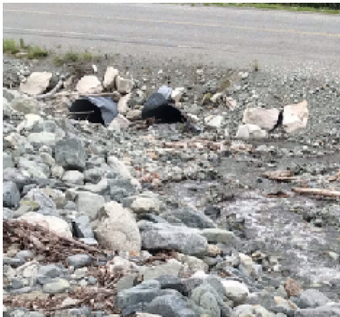
Figure 4 – East Culvert before MOTI work
