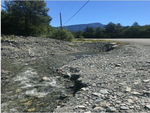
Figure 2 – East Culvert (June 2021)
