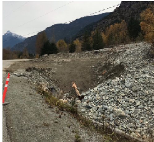
Figure 5 – MOTI work clearing East Culvert
