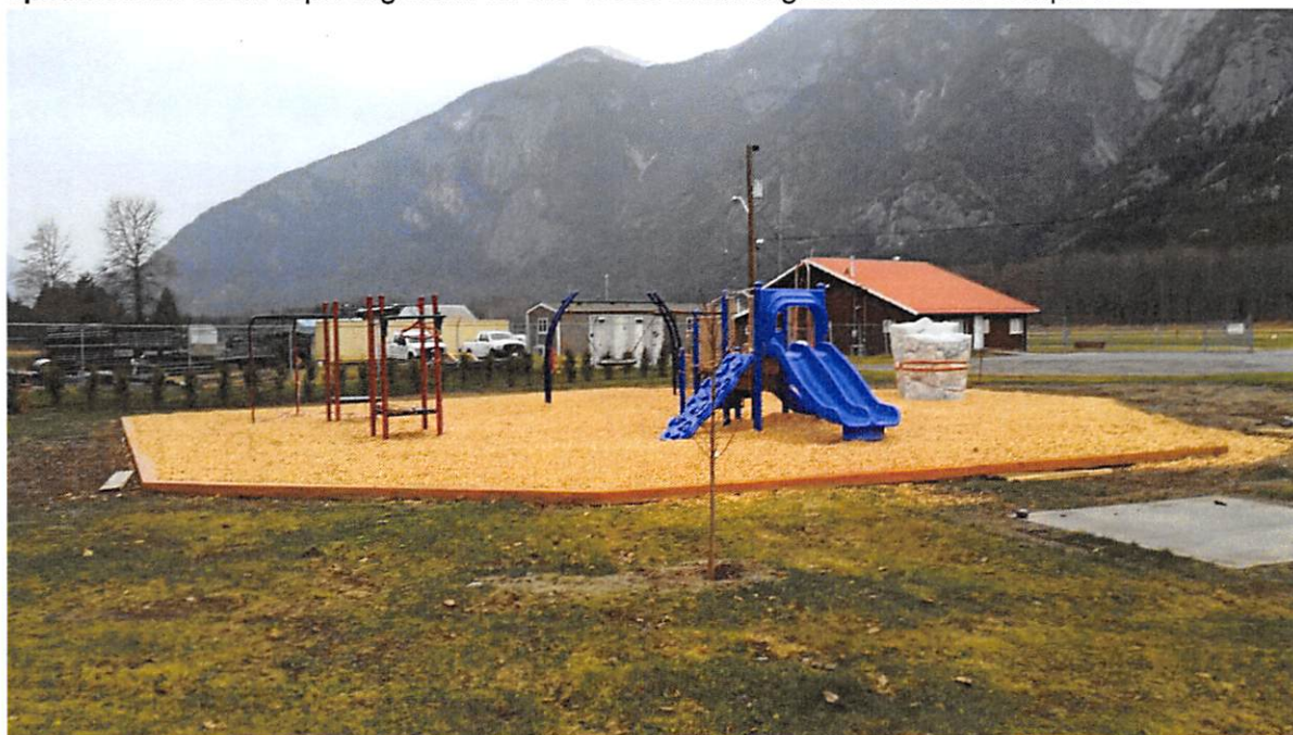
Photo: Engineered wood chips certified to meet CSA standards for playground use have arrived and been installed in the new play area.
