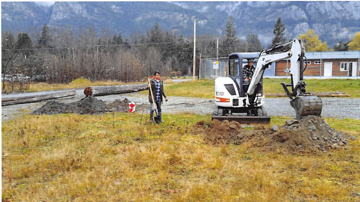
Photo: Geotechnical Engineer Hamid Tavakolian Bana records soil information from six test pits on site.
