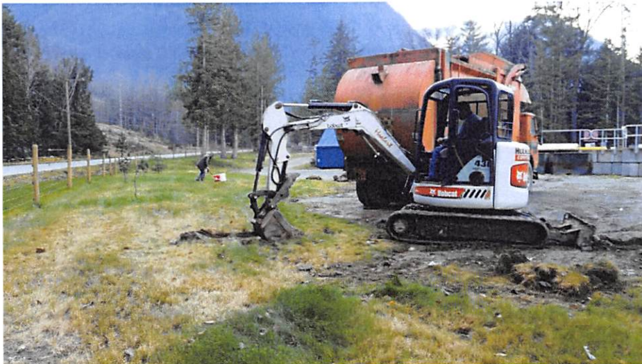
Photo: Digging test pits for percolation tests.
