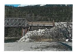
The project will replace the two wooden spans at the south end of the bridge (shown here) with a single-span concrete girder that will connect to the 180-foot metal section. The improved crossing will serve safety and reliably for decades to come.
