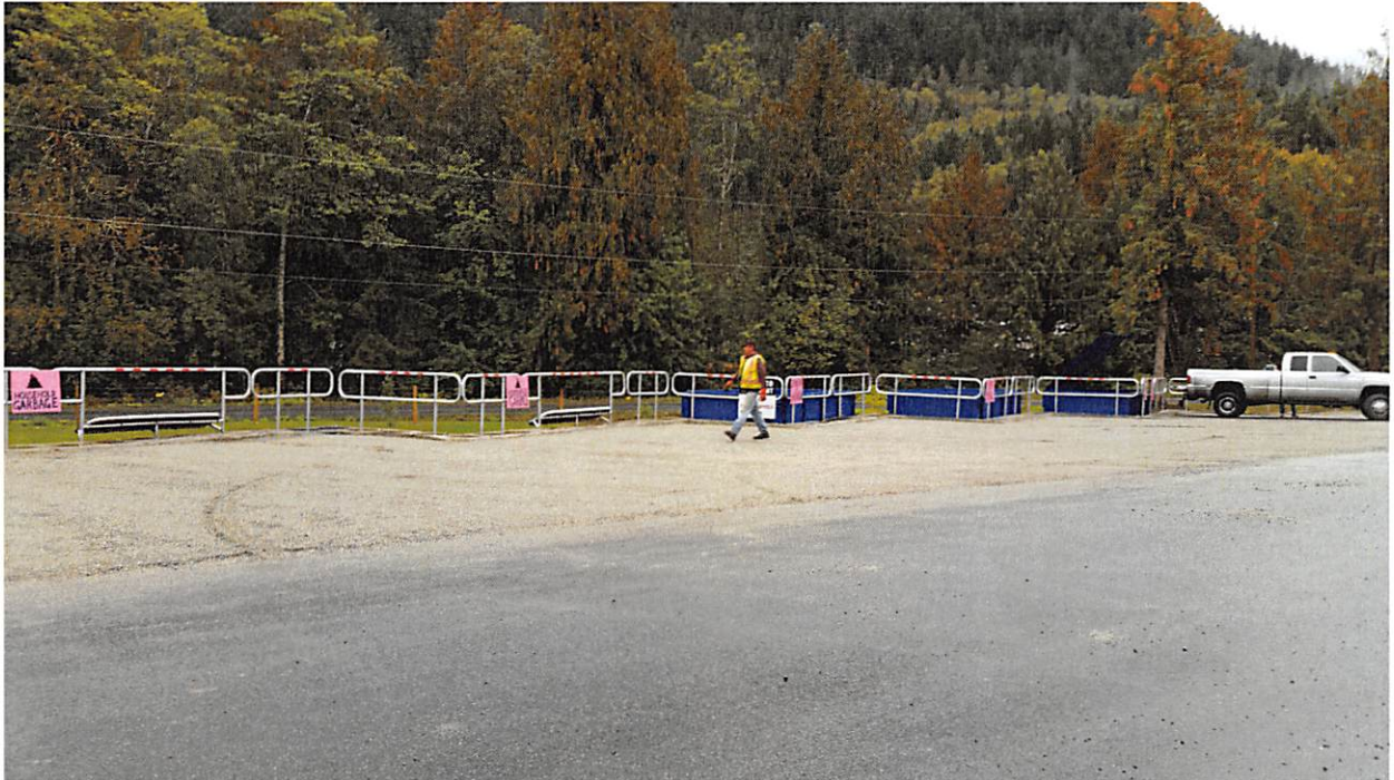
Photo: New drop off area for household garbage, metals, construction debris and wood waste.
