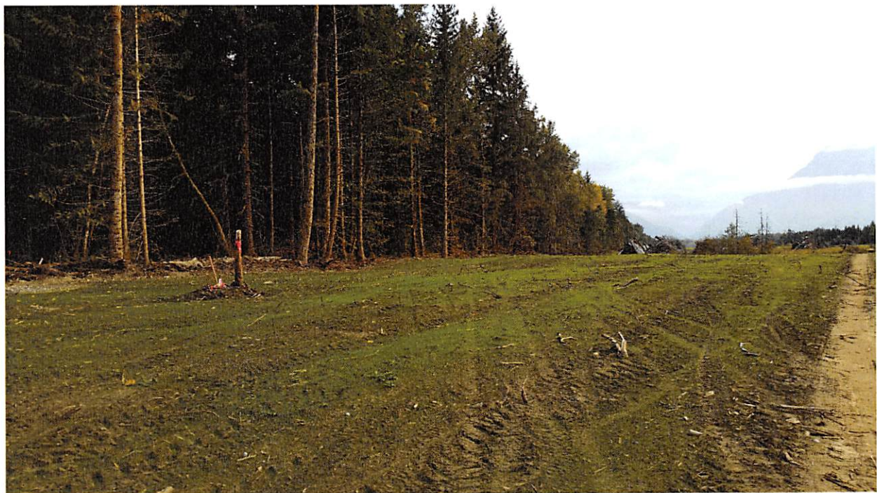
Photo: Private land portions on the northwest end have been cleared, raked, rotovated and seeded.
