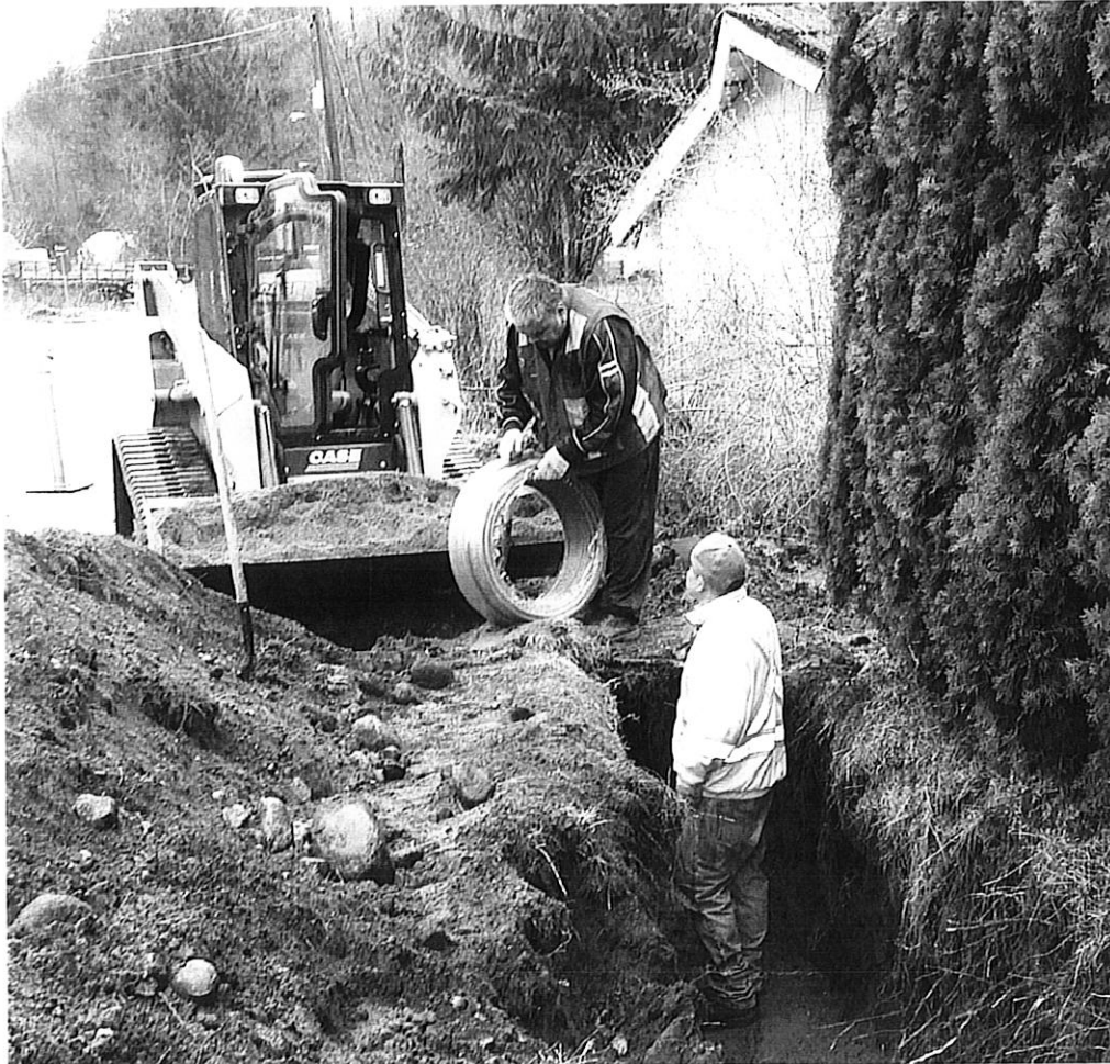
Photo: Nuxalk Band employees Brad King and Lorne Moody installing waterline.
