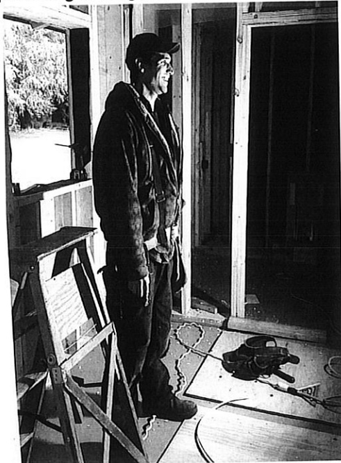
Photo: Electrician Max Anderson roughing in electrical.
