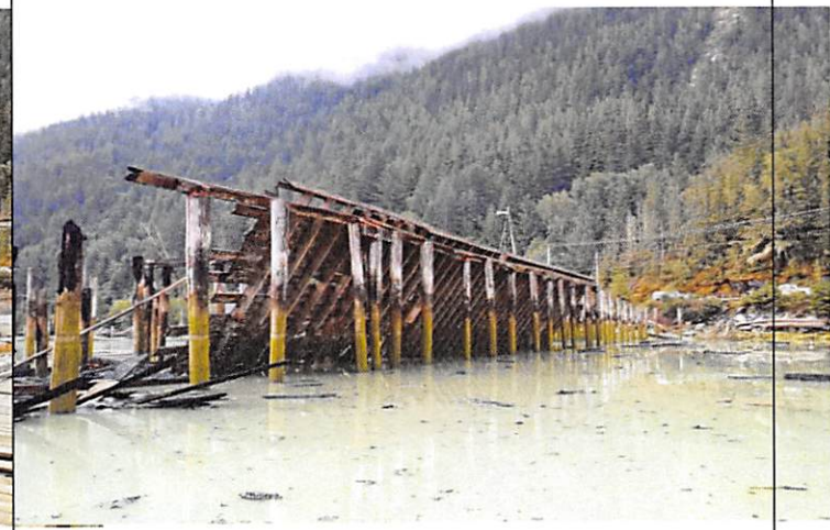
Photo 4: walkway and approach to the building area. Burned and partially collapsed approach leading from the shoreline to the burned building site.
