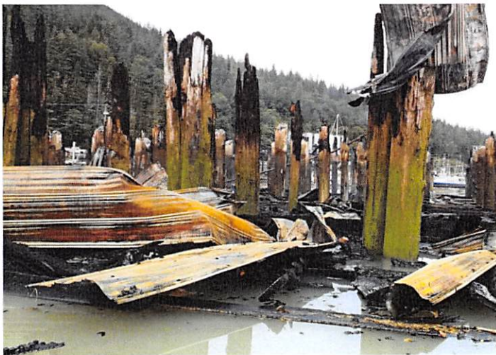
Photo 7: Metal roofing debris beneath collapsed/burned structure.
