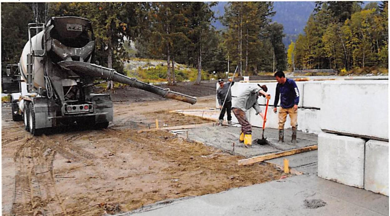
Photo: Concrete bin pads at new TCWRC Transfer Station
