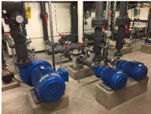
Three-phase, base-mounted centrifugal pumps will be used for the filter pumps and warming pool jet pumps. The pumps will have a protective coating to prevent corrosion from the chlorinated pool water. The pumps will be supplied with VFD's and controlled via a turbidity meter. The speed will range from design flow rate to BC health code minimum flow rate. The adjustable turbidity level will be set to maintain a 0.1 to 0.5 NTU (nephelometric Turbidity Units).
