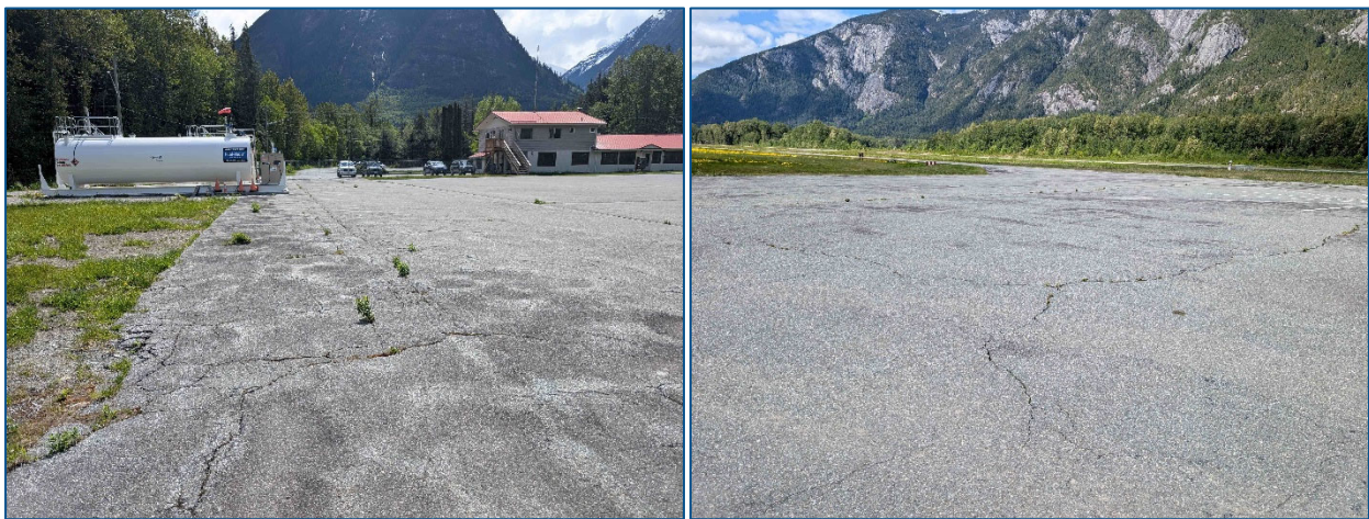
Pavement Repairs (left) and Recessed Aircraft Tie-Down Anchors (right)
